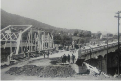
A 1937 image showing the construction of the new concrete bridge in the foreground with the old steel bridge in the background. This photo was taken from the intersection of Main Street and Parkway Drive looking towards the Pattonsburg neighborhood.
